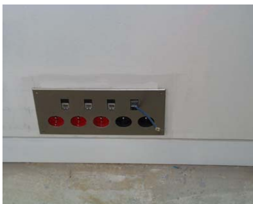
Workstation (worksite phase)
